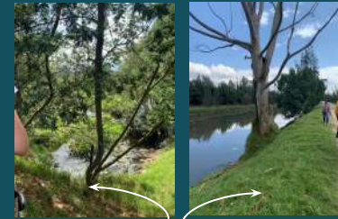
Bogota river and earthen flood levees ... cuts off the exchange between the wetland and the river at Humedal Jaboque
